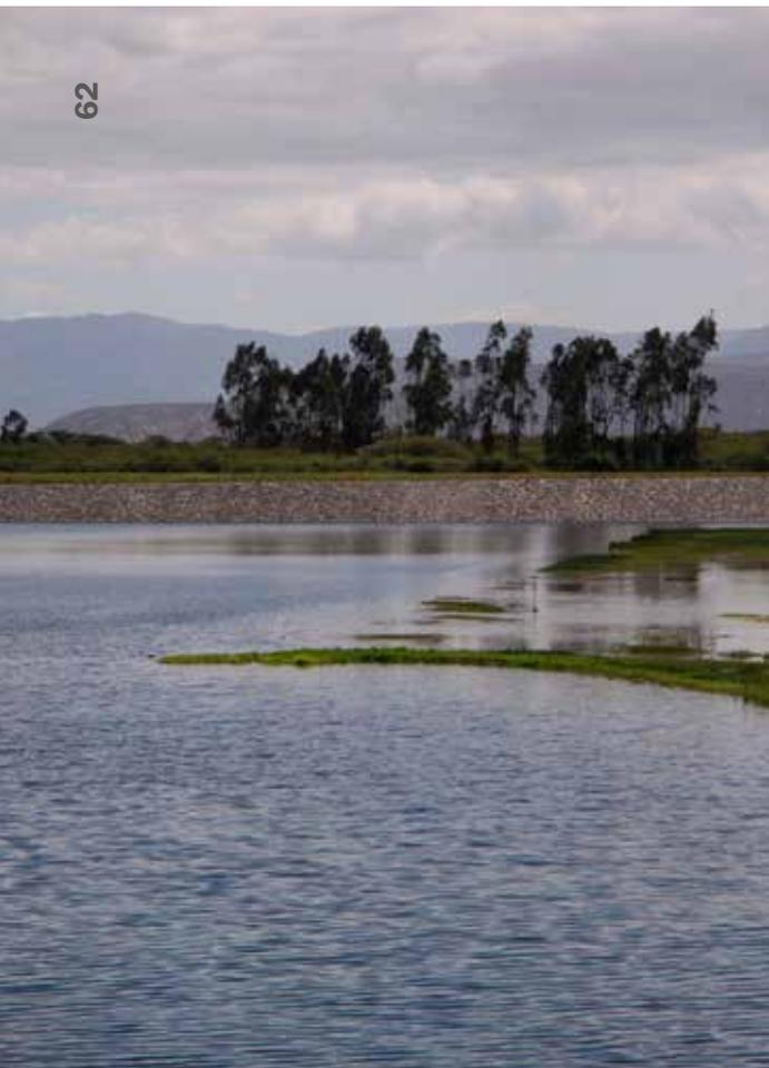
The reservoir of the Mariscal Sucre International Airport regulates rain water to reduce wastewater discharge and provides a resource for construction activities and fire response.
